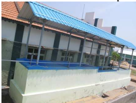
Indigenously designed biofilter system for broodstock tank
