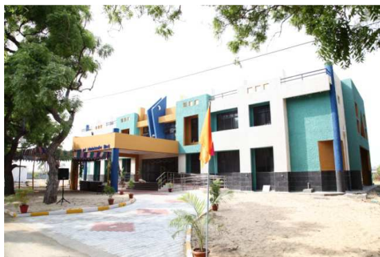
View of Research and administrative block
