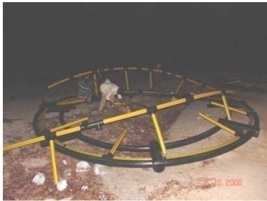
Fabrication of sea cage
