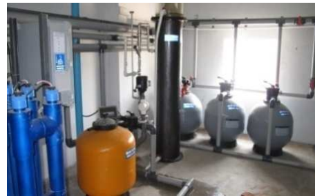
Imported RAS components (UV filter, Bead filter, Protein skimmer & Reactors)
